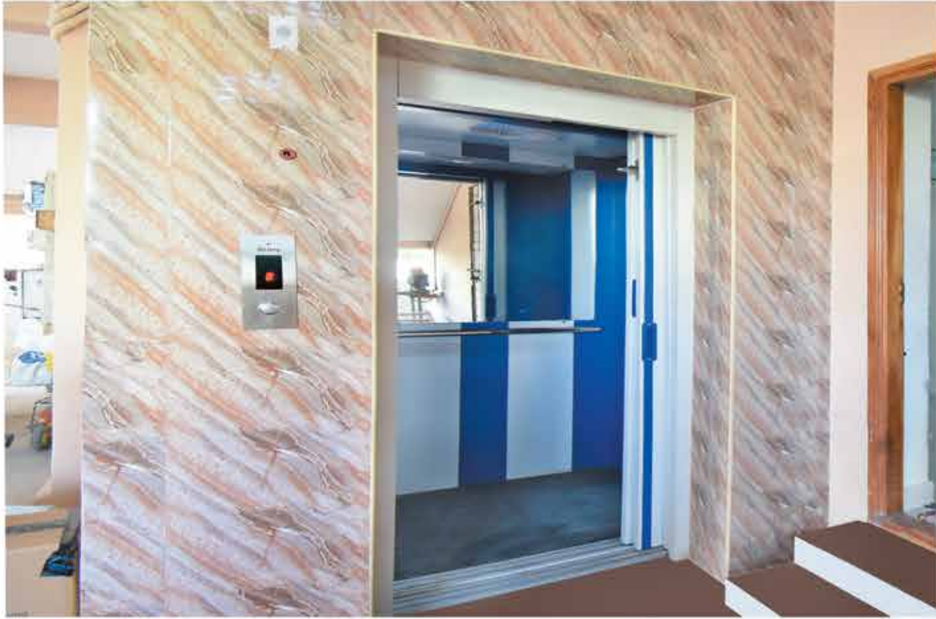
M.S. Cabin with Manual Sliding Door
